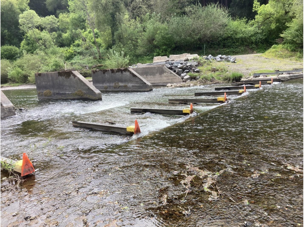
Figure A 3. Looking across the Vacation Beach dam sill on April 13, 2022.
