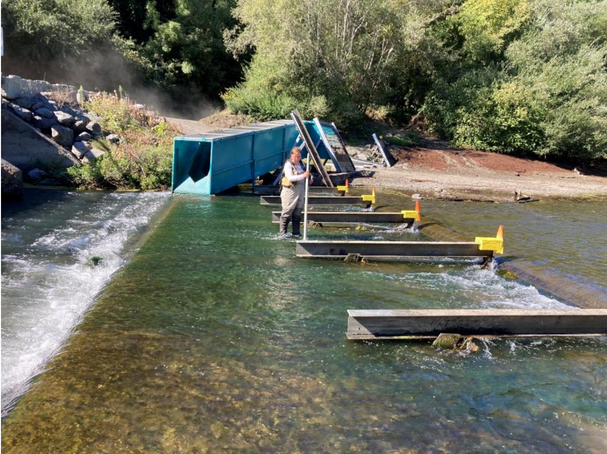
Figure A 13. Looking across the Vacation Beach dam sill on September 30, 2021.
