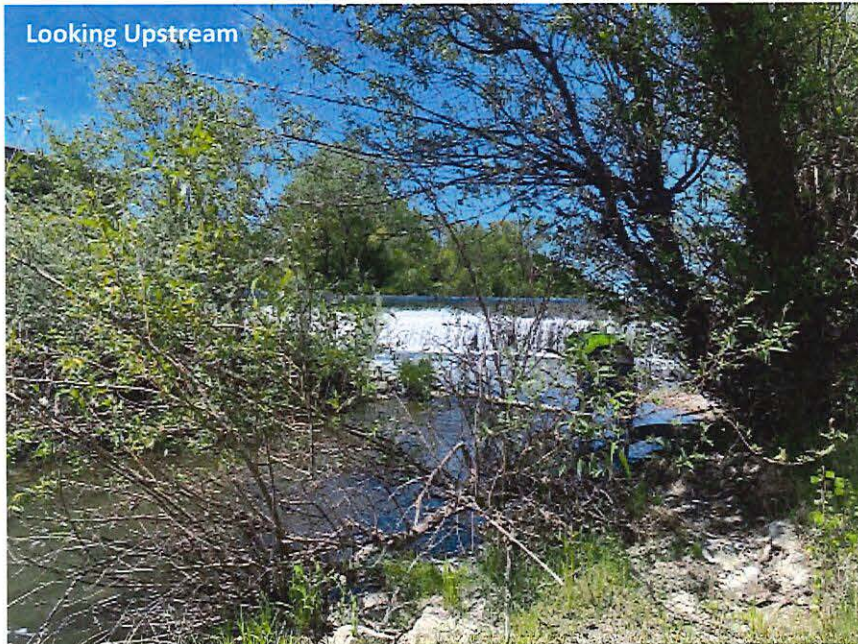
Mirabel Inflatable Dam
