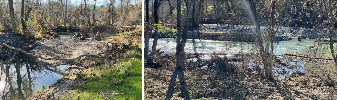
The photograph on left depicts sediment deposition at the inlet of Site 4C, which is a backwater channel constructed in 2024, that will obstruct the inlet at lower flow. Downstream connections between the mainstem and the channel remain open. The photograph on the right depicts the mainstem (background) filled in with sediment and avulsed into the newly constructed Site 2B backwater channel (foreground). Both photographs were taken in January 2025.
