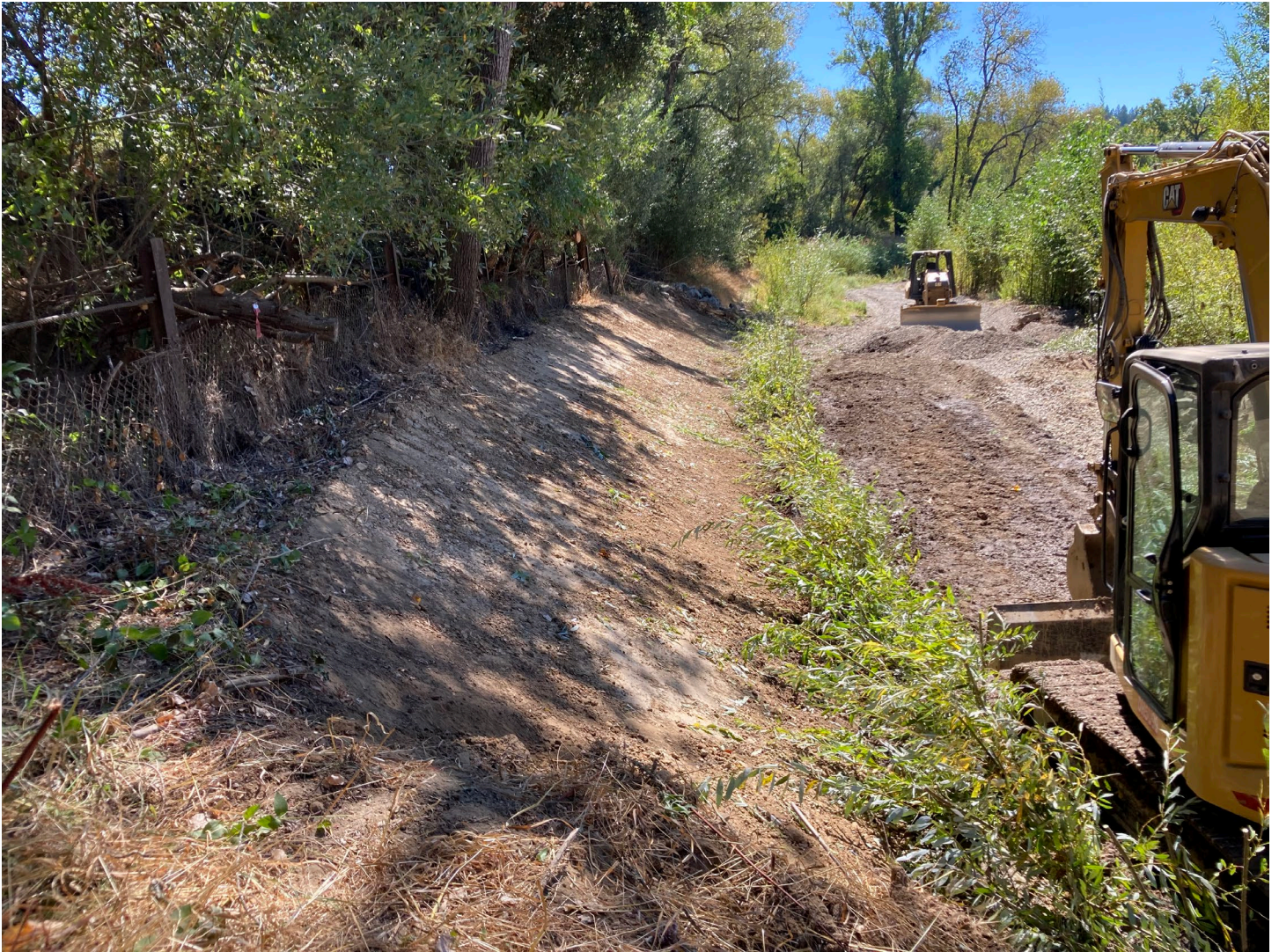
Photo of eroded bank of habitat channel stabilization work. Photo shows regraded bank slope, new willow cuttings at the toe of the slope and excavation of the habitat channel area. Photo taken September 26, 2024.
