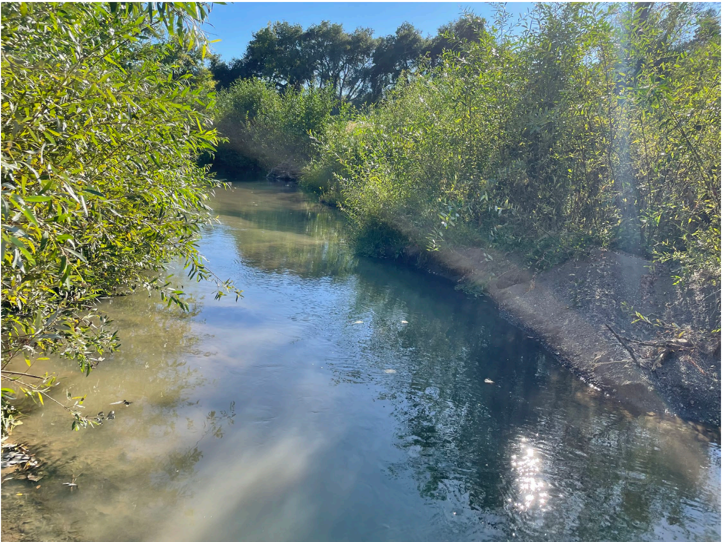
Photo of the lower portion of the habitat channel in Reach 5A where flow was recently restored back into. Photo is looking downstream along the constructed habitat channel in Reach 5A. Photo taken October 9, 2024.
