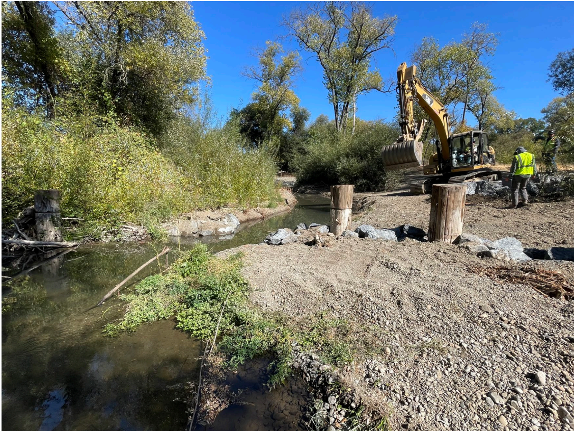
Photo of newly opened portion of the habitat channel. Photo is showing the inlet connection from Dry Creek into the habitat channel in Reach 5A. Photo taken October 3, 2024.
