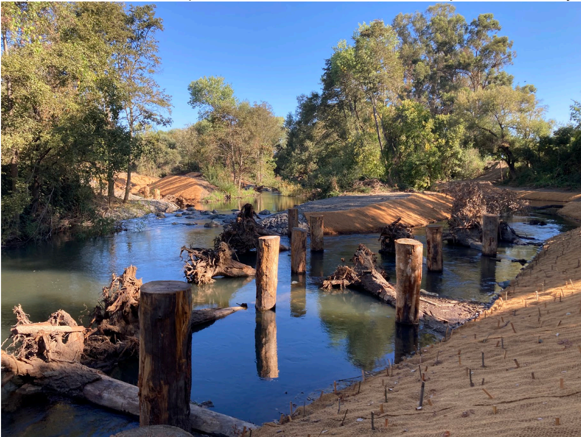
Reach 2 sites on September 4, 2024. View is looking back upstream with the main channel of Dry Creek in the center and a newly constructed side channel visible on the right and the outlet of a newly constructed side channel visible to the left of the main channel.
