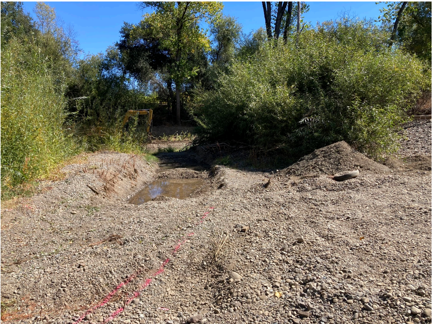
Photo showing portion of the Reach 5A Channel that had filled in. Habitat channel shown is in process of being re-excavated. Photo taken September 26, 2024.
